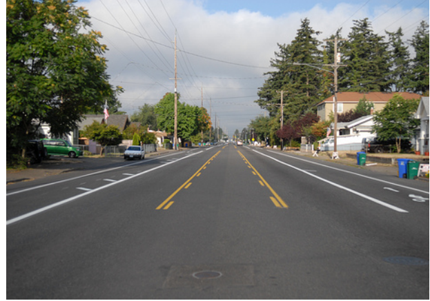
One-way Bicycle Lane on each side of side with reversible centre lane in Portland ( http://www.bikeportland.org )
