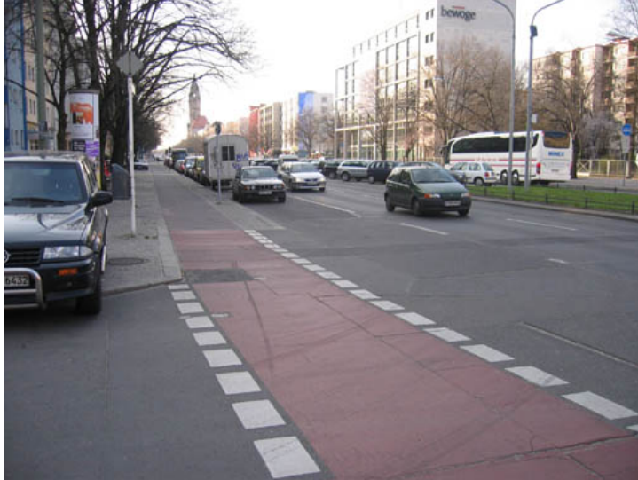
Cycle track in Berlin transitioning into a coloured bike lane at an intersection ( http://www.planetizen.com )
